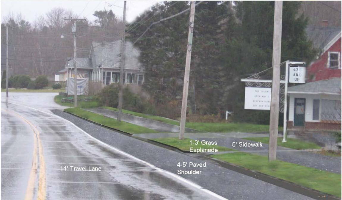
**Figure 5 Conceptual Illustration of Sidewalk, Esplanade and Shoulders in Hulls Cove**
