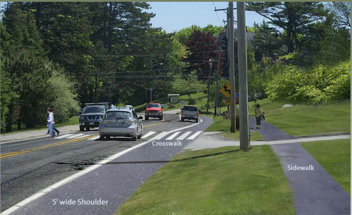
Sidewalk to Service Motel/Hotels Across from College of the Atlantic
