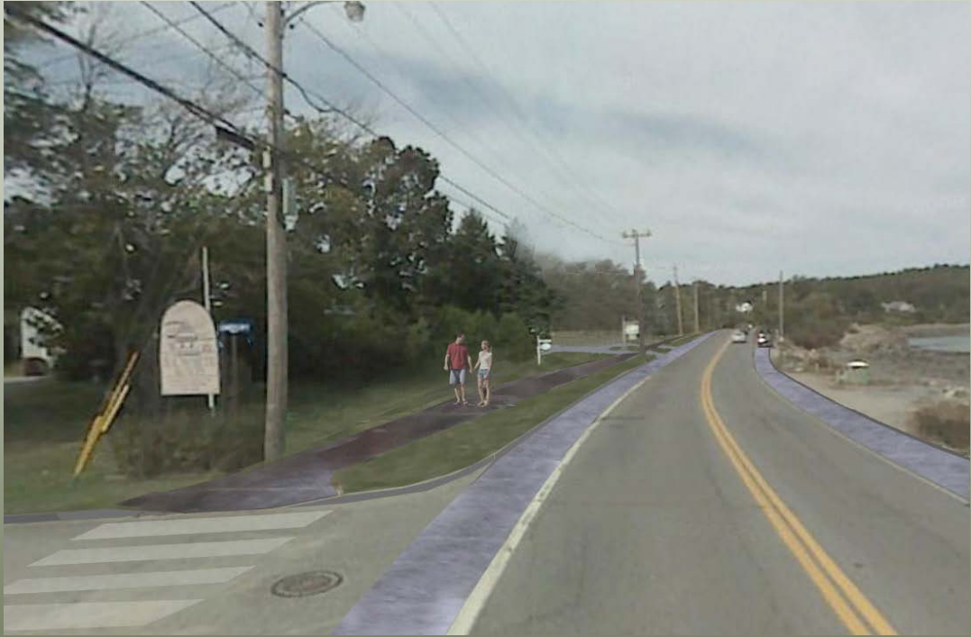
Hull's Cove Sidewalk to Service Colony Motel
